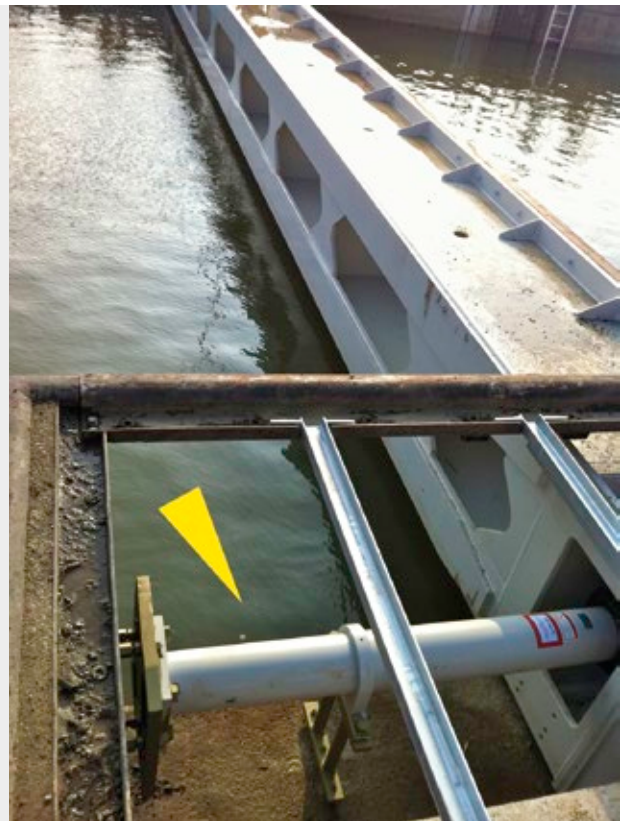
Heavy safety shock absorbers, which are specially designed for this application, are able to brake in lock masses of up to four million kg Mourik Limburg BV, 6101 AJ Echt, Netherlands
